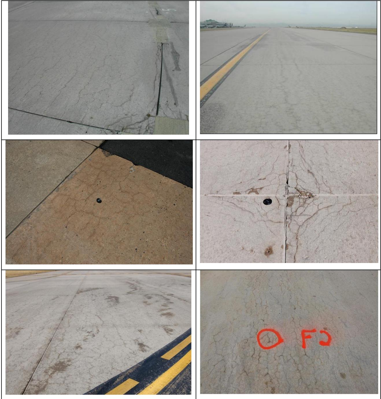
Figure 1 – Typical Patterns of Deterioration in Six Different Airfield Pavements Exposed to Deicing Chemicals
