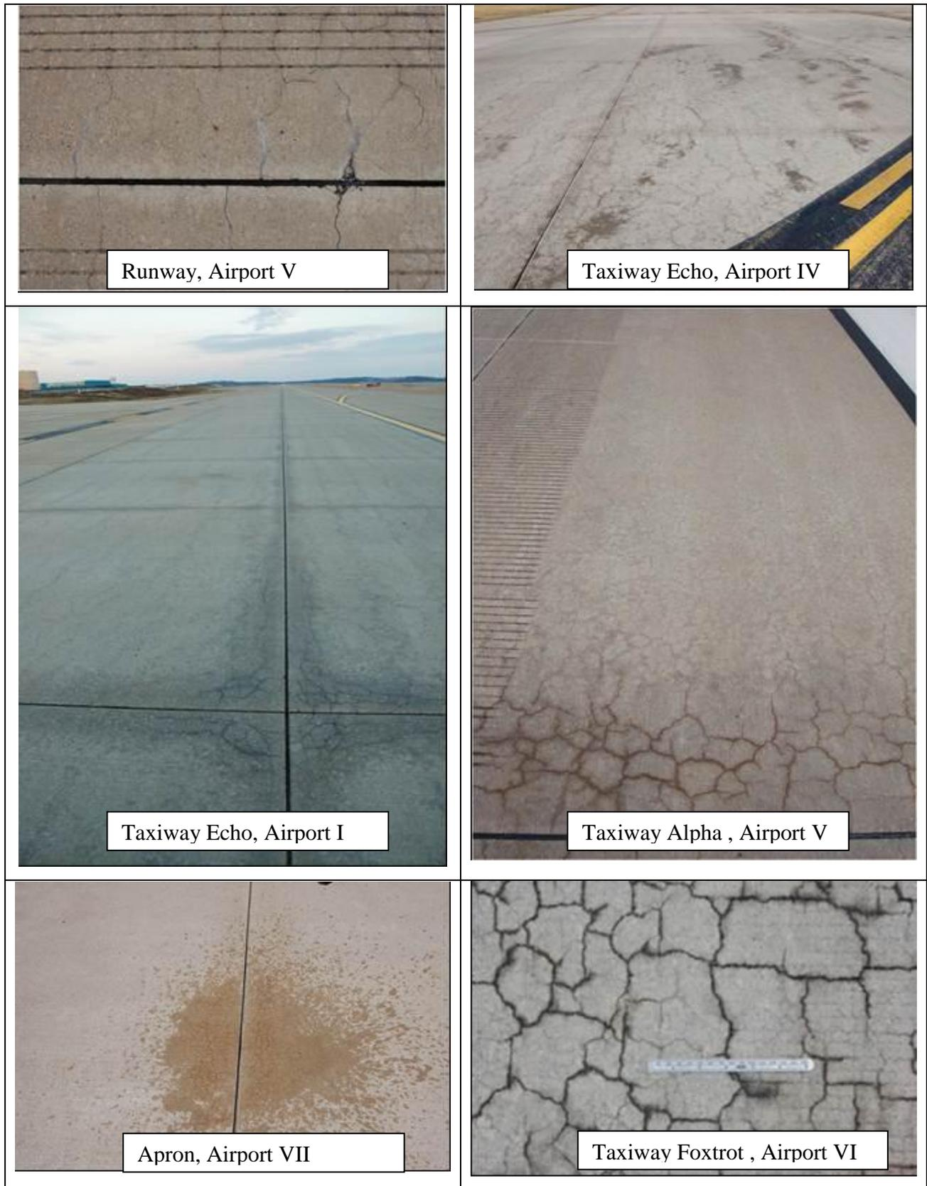
Figure 2B – Typical Deterioration in Airfield Pavements
