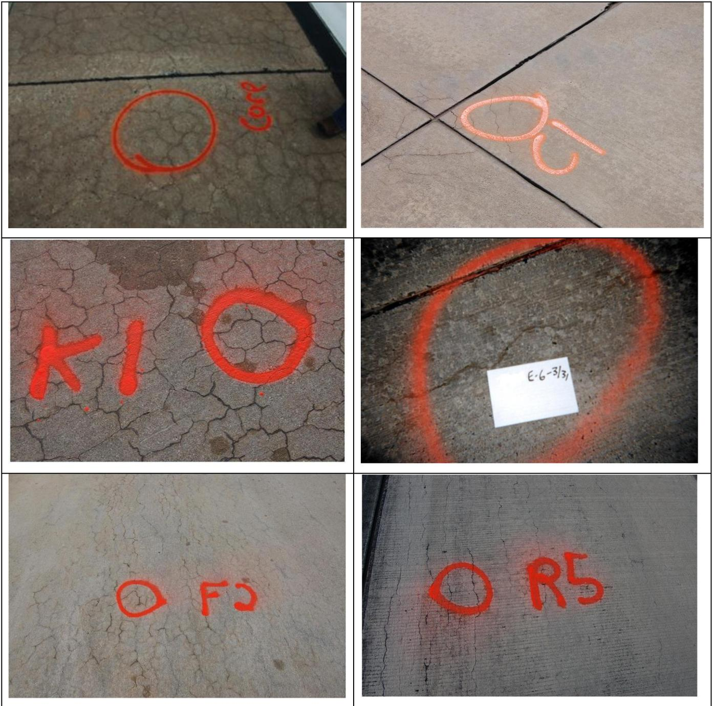
Figure 4 – Typical coring locations in airfield pavements to capture distress of different intensity
