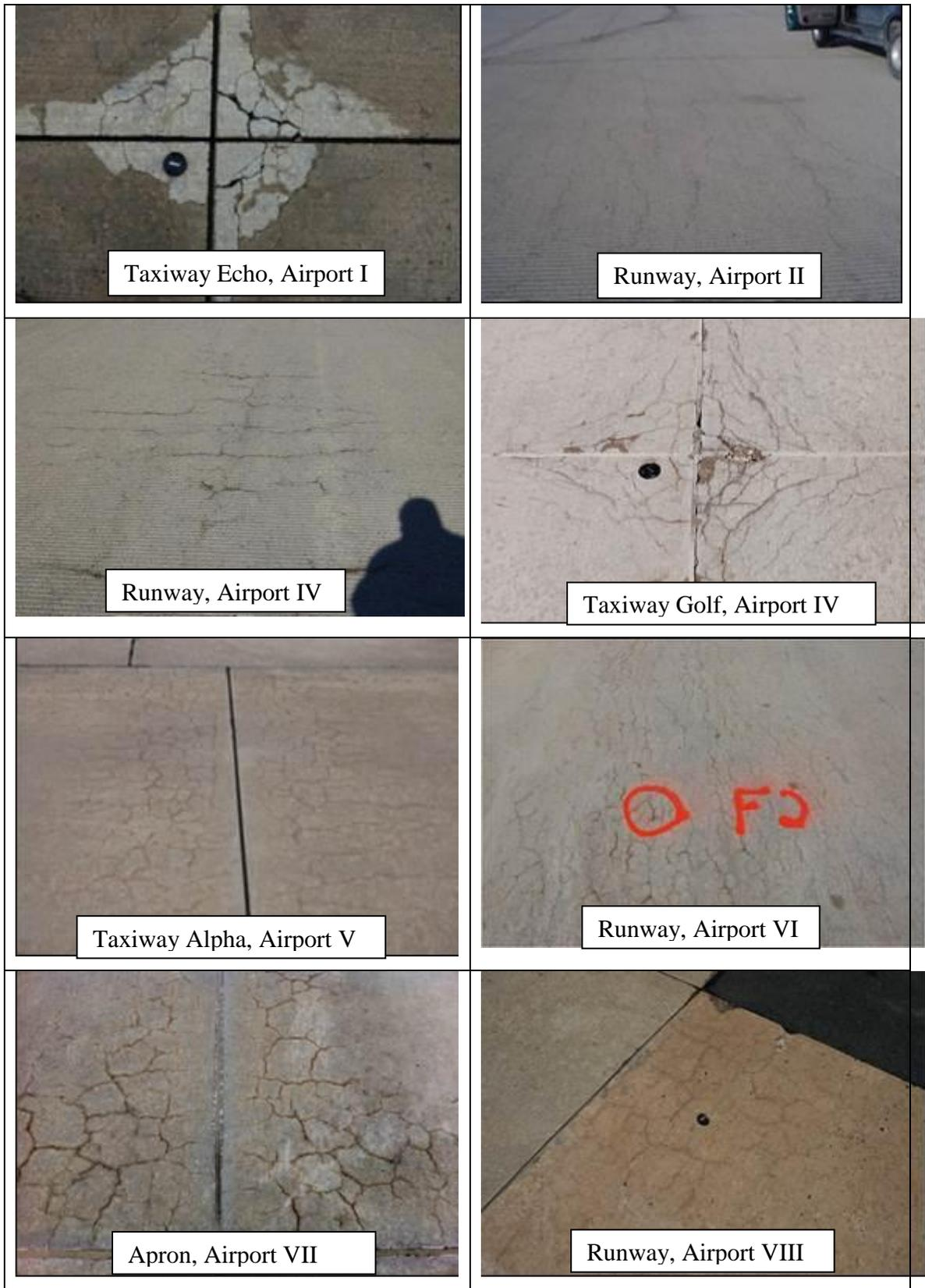
Figure 2A - Typical Deterioration in Different Airfield Pavements
